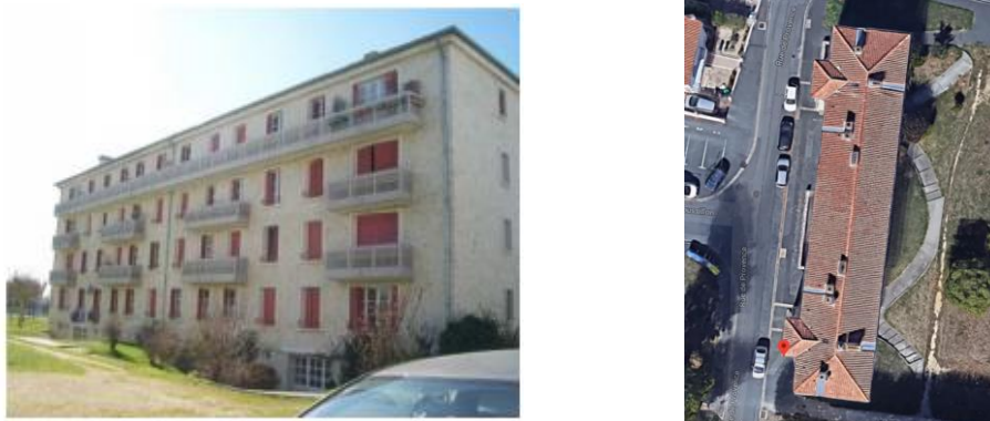
Figure 44: PN6 Building East façade and roof
