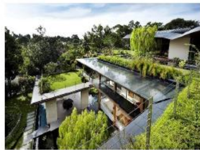
Green roof/ roof pond
